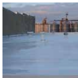
2. Prime surface with Tack Coat™.
