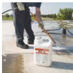
1. Power wash and clean with Wac™ II Roof Cleaner.
