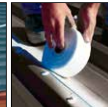
Reinforce existing seams with SpunFlex™ or Butyl Tape and base coat.
