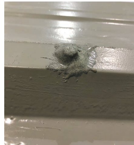
Acclaim® FSG applied by chip brush over fastener head on an R-panel metal roof system prior to coatings application.
